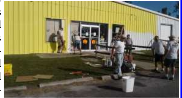
Spraying Yellow Final coat of paint over white primer.
